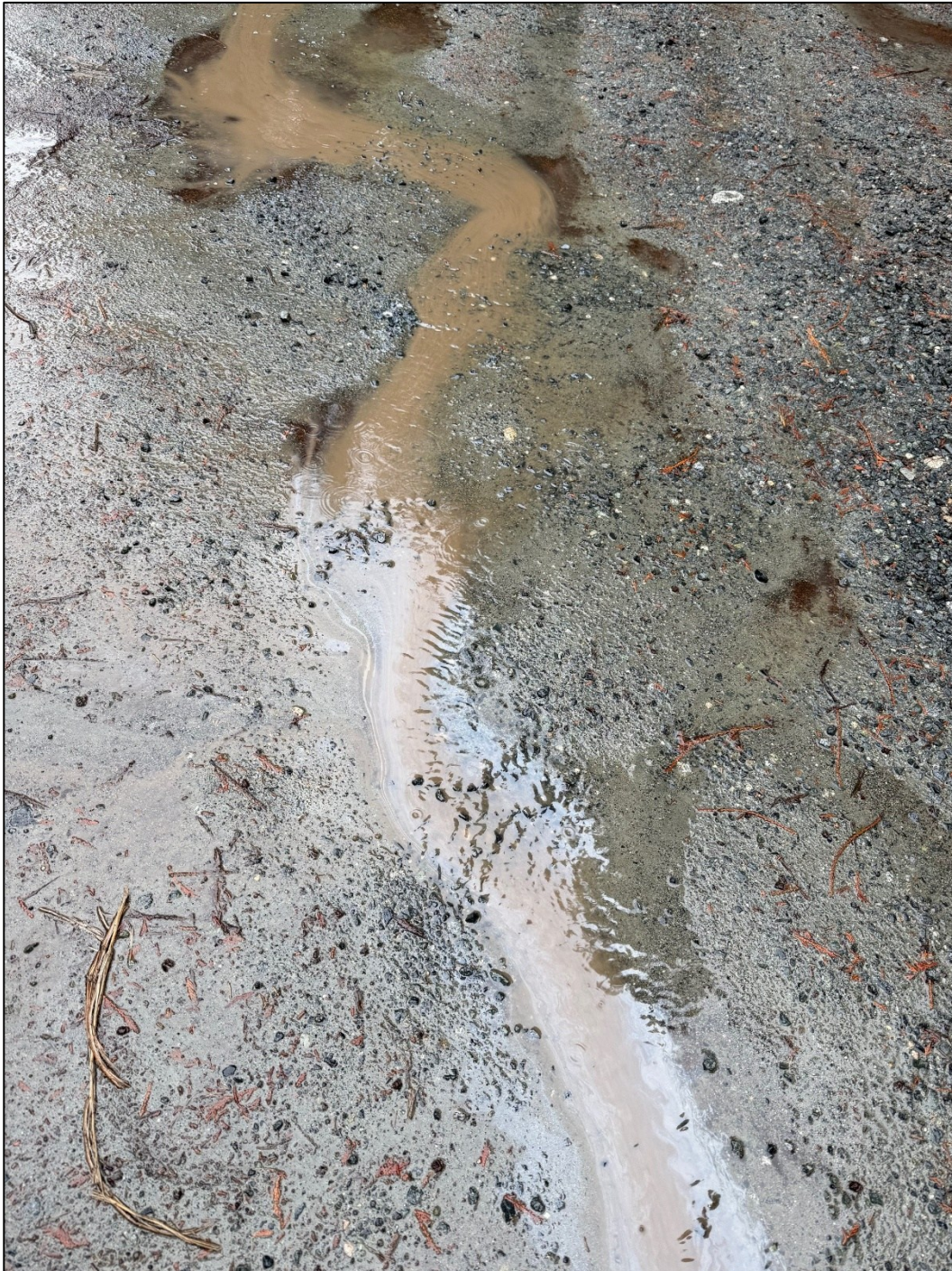
Photo 1: Oil runoff down the Duck Lake boat launch.
