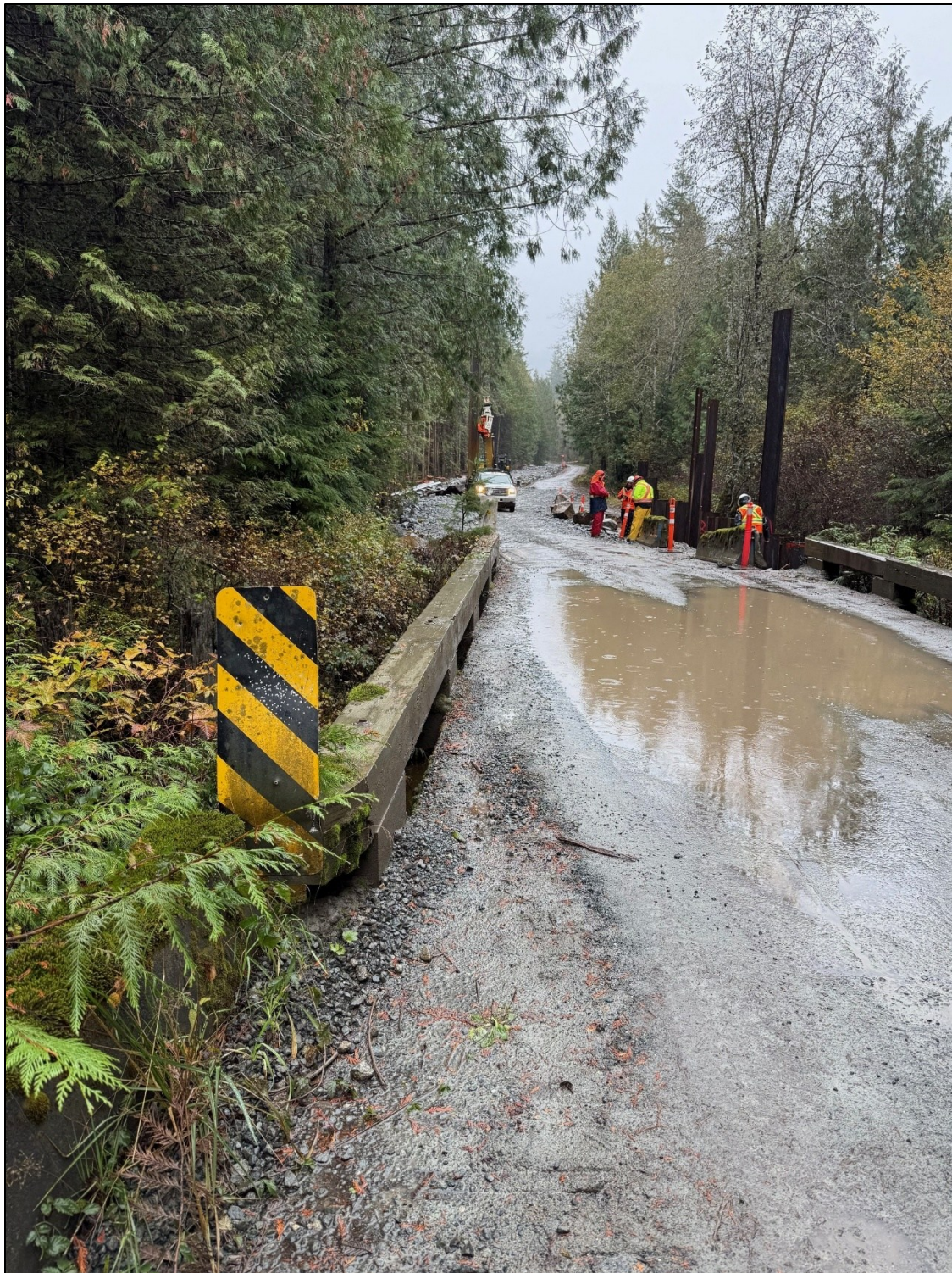
Photo 2: Blackwater Creek bank armouring and road shifting work.
