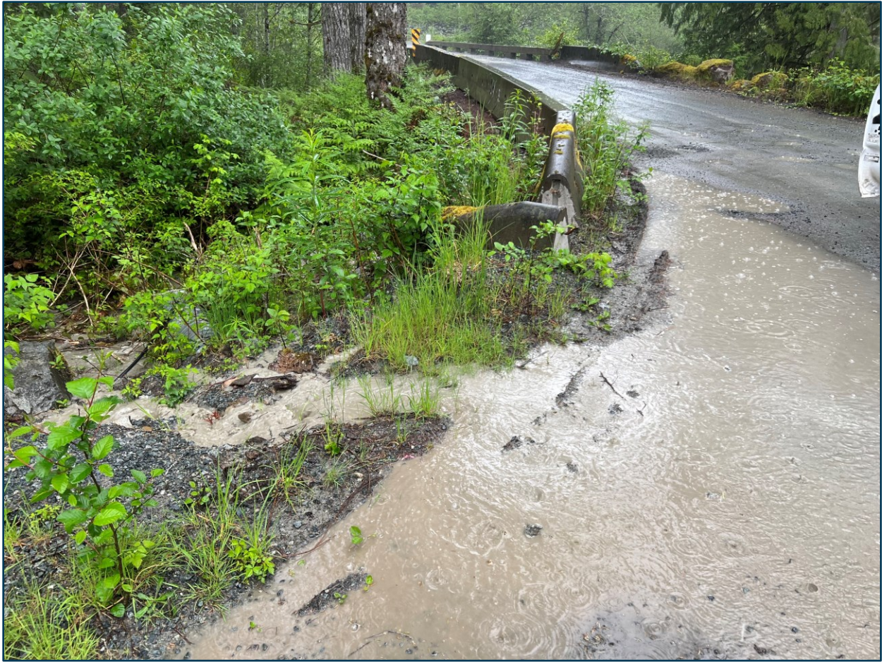
Photo 2: Sediment-laden water flowing into Duck Lake from a road. Photo taken on June 3, 2022.
